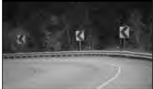
Figure F-4. Chevron Signs on Outside of Curve
